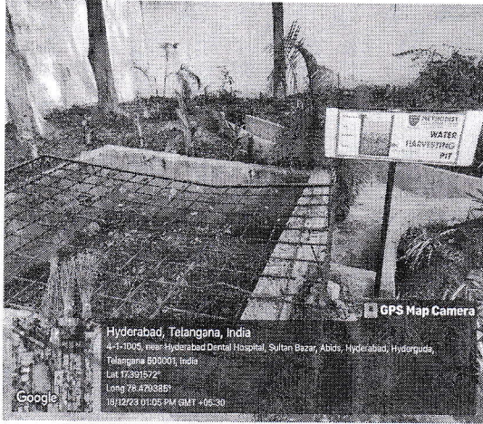
Water Harvesting PIT-1 near E Block
